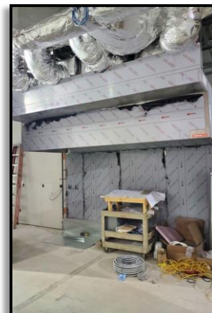
Deli Hood Installed
