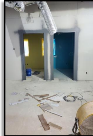
Office Area Painting
