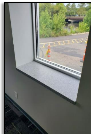
Window Sills Installed
